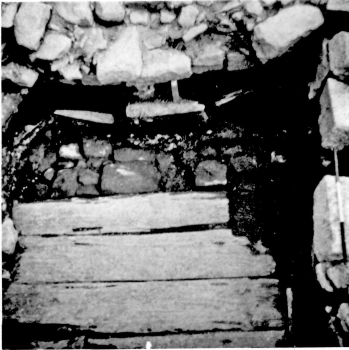
Fig. 8. (2E-1289 X) View of the east end of Room 2, 2E17G7, floor level. Note that planks of floor end at the edge of the earlier wall paralleling east barracks wall.
